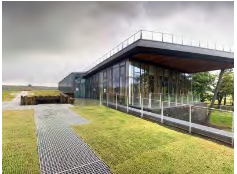
Part of the Sill roof as seen at an early stage in 2017. The coir matting can clearly be seen in the planted areas.
